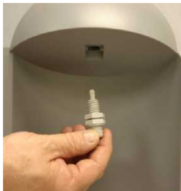
FIGURE I: DISS FITTING REMOVAL
